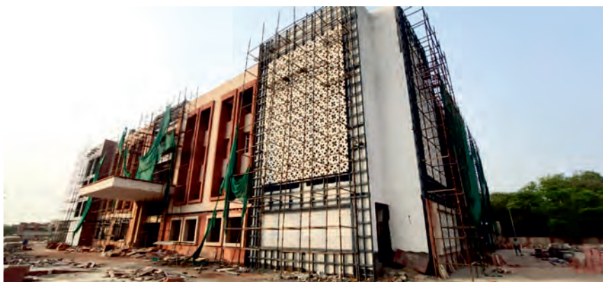
Construction work at new office building
